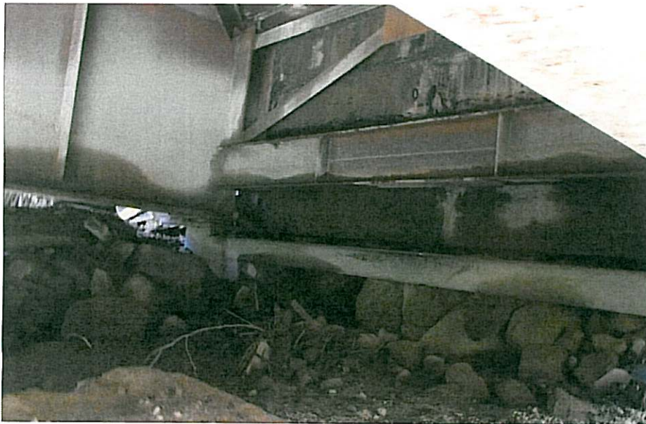
CK-2271 Left Abutment
