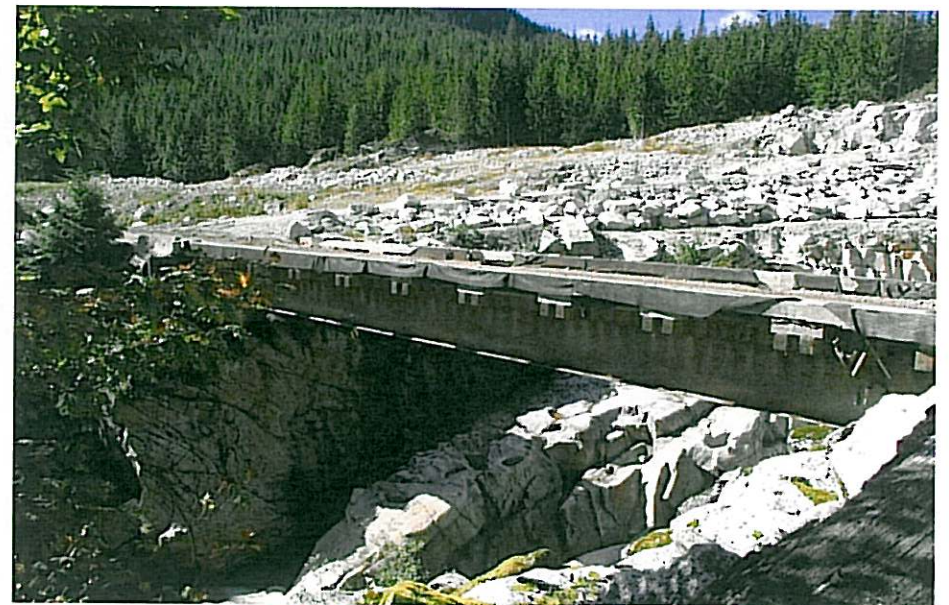
CK-2271 From Downstream (2)
