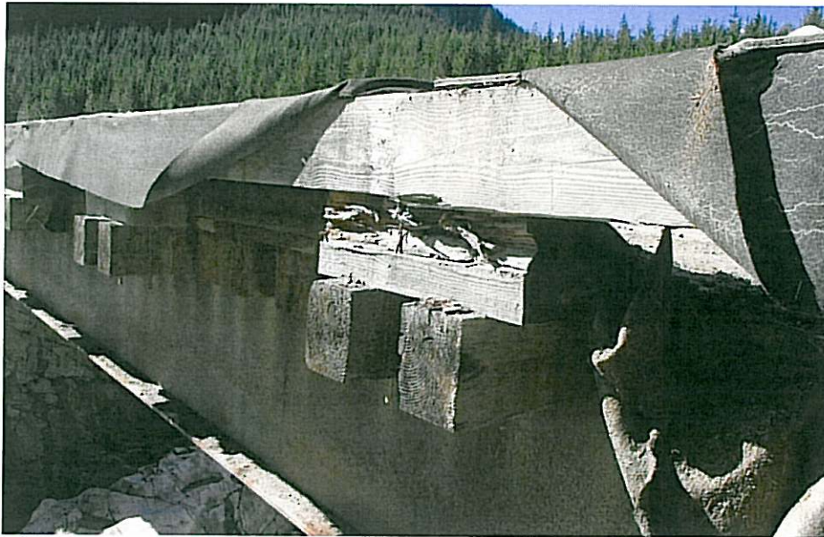
CK-2271 From Downstream
