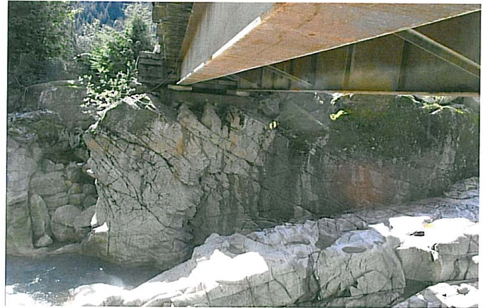
CK-2271 Right Abutment
